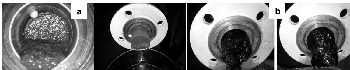
Figure 5. Cleaning of pipe from mechanical impurities and corrosion deposits (a) and from ARPD (b)
